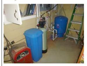
17. WELL PUMP / STORAGE TANK - The well pump is believed to be submerged in the well itself. The storage tank is located in the basement workshop. Both components are believed to have been functioning as intended at time of the inspection.
