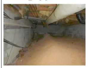
12b. / 14. / 17. PRIOR WATER INFILTRATION / SUMP PUMP / INTERIOR French DRAIN - A sump pump is located in the vault area beneath the front porch. The collection container was dry at time of the inspection with no indication of any recent moisture infiltration. The home owner indicated that an interior French drain had been installed in the vault area to work in conjunction with the sump pump. An evaluation of the pump itself is not offered.
