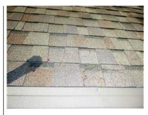
1b. SHINGLES - The Inspector did not observe any abnormal wear and tear or evidence of leak activity associated with the roofing shingles at time of the inspection other than that noted above. The home owner has indicated that the shingles were installed in 2010. 25 year wear rated architectural shingles have an average life expectancy of 20 to 25 years. The wear rating for the shingles observed at time of the inspection is not known, however, are at least 25 year rated.
