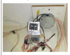
8c. GARAGE OUTLETS - The garage outlets are not GFCI protected as would be expected present day. The absence of GFCI protection is now considered to be a safety hazard. Upgrading to include GFCI protection of the subject outlets is recommended, however, should not be considered a requirement of the present owner.
